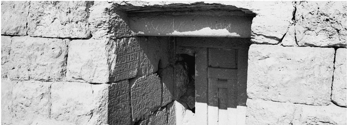
Fig. 13. G 2197, Penmeru, general view of chapel niche, including the undecorated false door, looking southwest. August, 1977. Photograph by Robert E. Murowchick, REM_1977.001.12.
